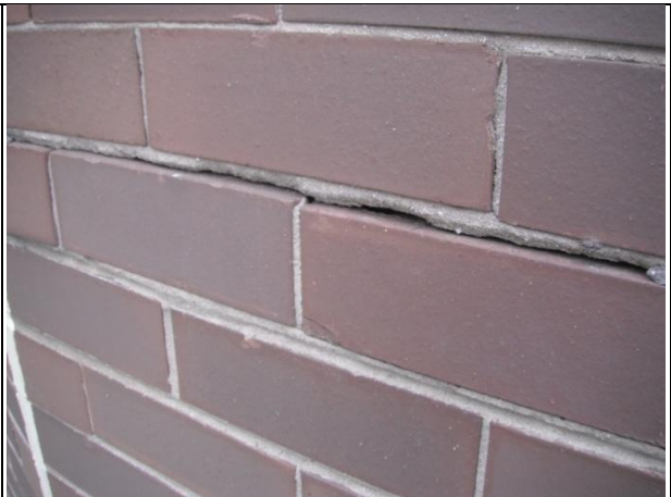
Ph #5518. Level 17. Horizontal Brickwork Crack
