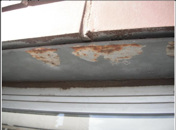
Ph #5487. Brickwork lintel onset of surface corrosion.
