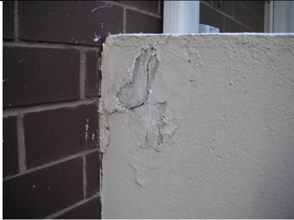
Ph #5471. Level 15. Cracking in render
