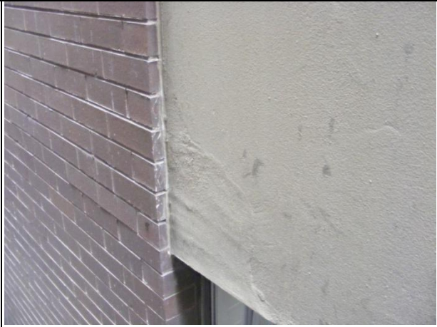
Ph #8740. Level 6. Extremely Drummy
