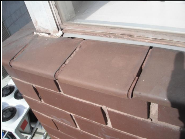
Ph #5493. Level 16. Loose window sill tile
