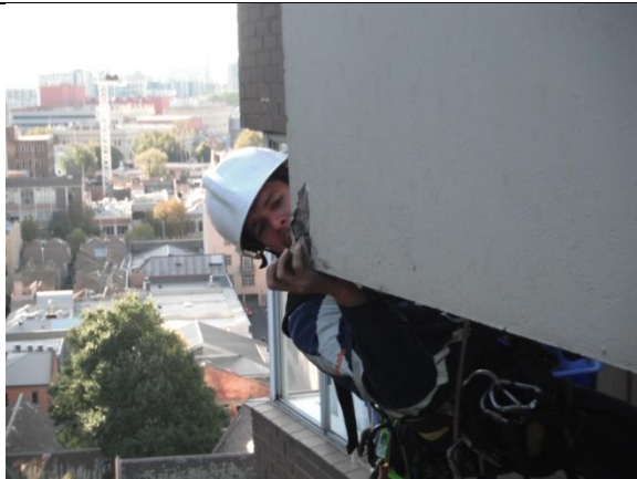
Ph #5471. Level 15. Cracking in render
