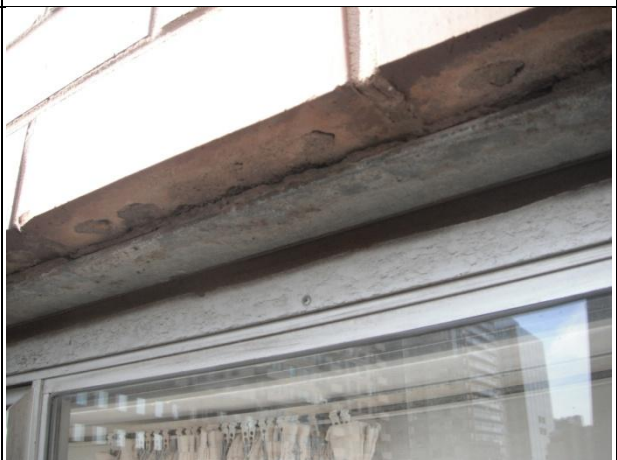
Ph #5487. Brickwork lintel onset of surface corrosion.
