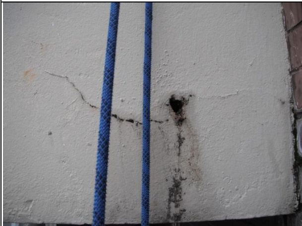
Ph #5184. Level 17 Drummy Render. Plant growing out of render
