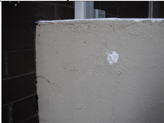
Ph #8561. Level 14 Cracking & loose render in lower corner balcony
