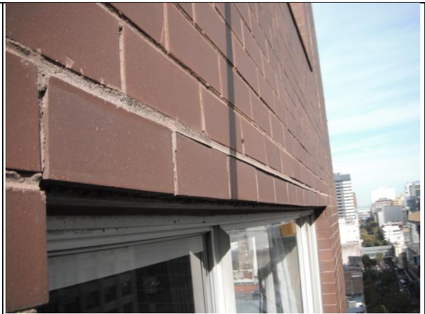
Ph #8573. Lintel Level 16
