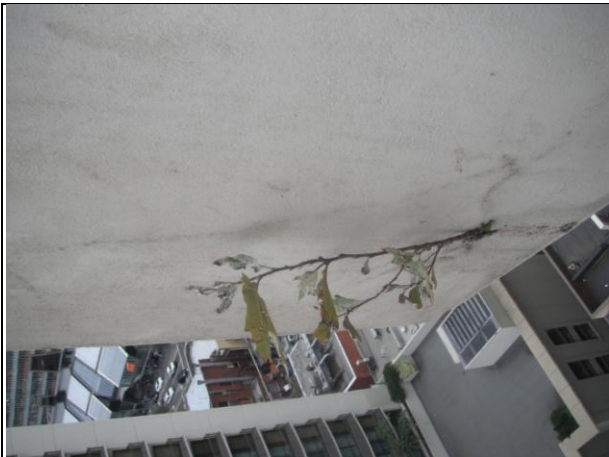
Ph #5184. Level 17 Drummy Render. Plant growing out of render
