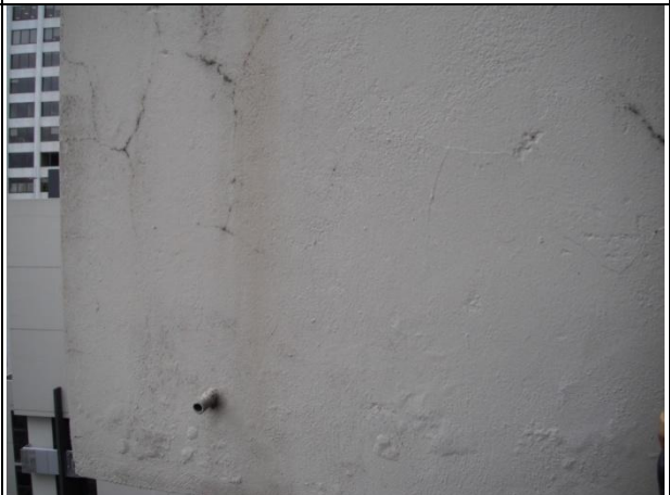
Ph #5518. Level 17. Horizontal Brickwork Crack
